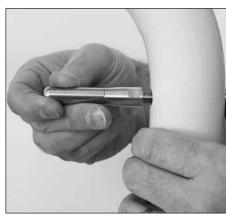
2. Thread the Push-Lock<sup>®</sup> coupler onto the post and tighten with 7/16" wrench.
