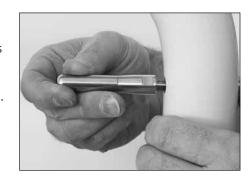
Thread the Push-Lock<sup>®</sup> coupler onto the post and tighten with 7/16" wrench.
