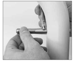
**3.** Pull the cable tightly along the side of the fitting and mark the cable 1-3/16" from the end of the fitting opposite the post. Mark and cut the cable on your mark.
