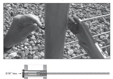
The swaging stud will be pulled into the Receiver by rotating the Receiver clockwise.
